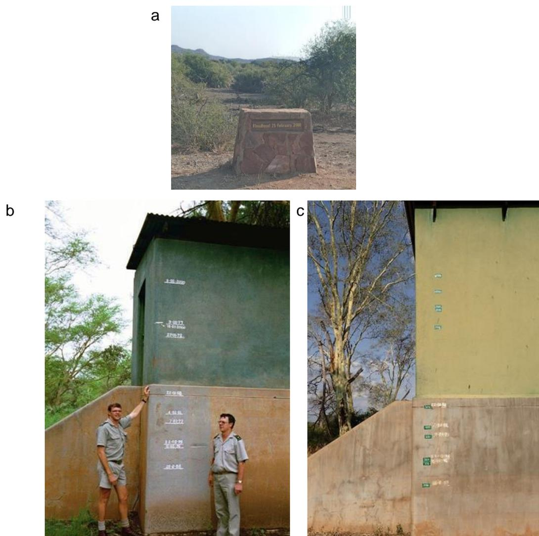
**Figure 4.14: Marked historic floods levels: a) (February 2000) - on beacons on the tar road crossing the Luvuvhu River, b) marked on a wall at the Theba Pump House between 1958 and 2000<sup>34</sup> - date unknown, c) includes the 2013 flood that is the second highest recorded after 2000 (photograph October 2022)**
